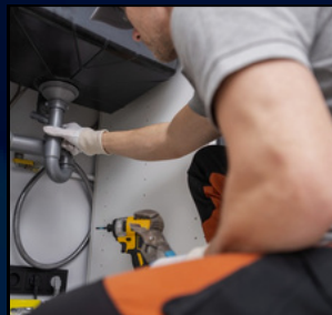
Cert II Plumbing Services 11054NAT
